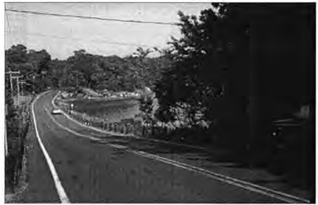
Figure 34 - Parking at the side of the road near water is a problem.
