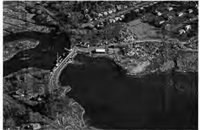
Figure 36 - Aerial view of the Montowese Street Bridge under construction at the Branford River.
