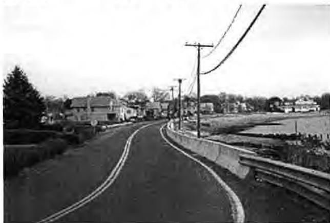
Figure 56 - existing Jersey barrier at Limewood Beach.
